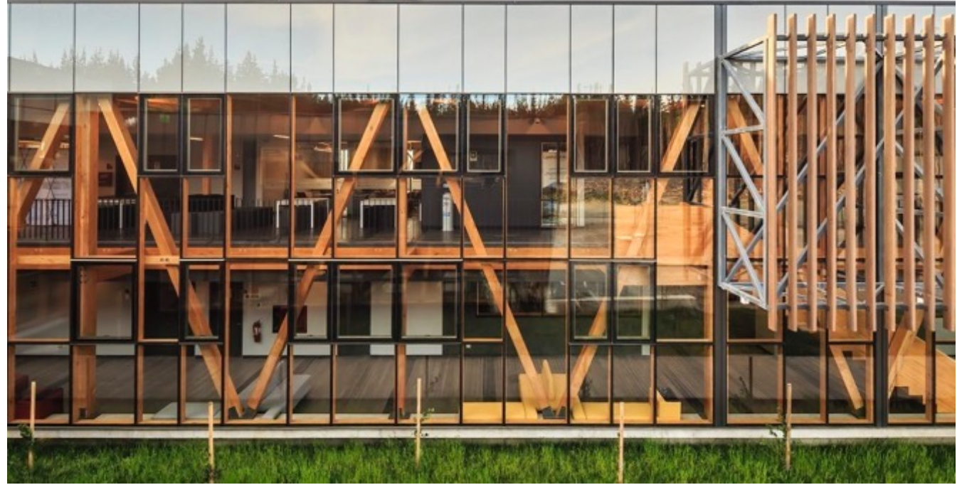
CFT ARAUCO DUOCUC / GDN Architects. Chile.
